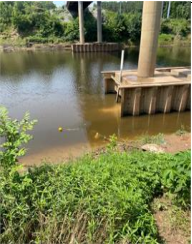
Reset sample inlet tubing and pipe
