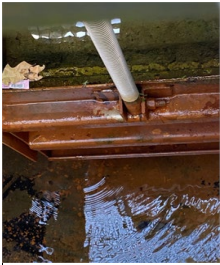
Inside effluent cell, just a drip of flow
