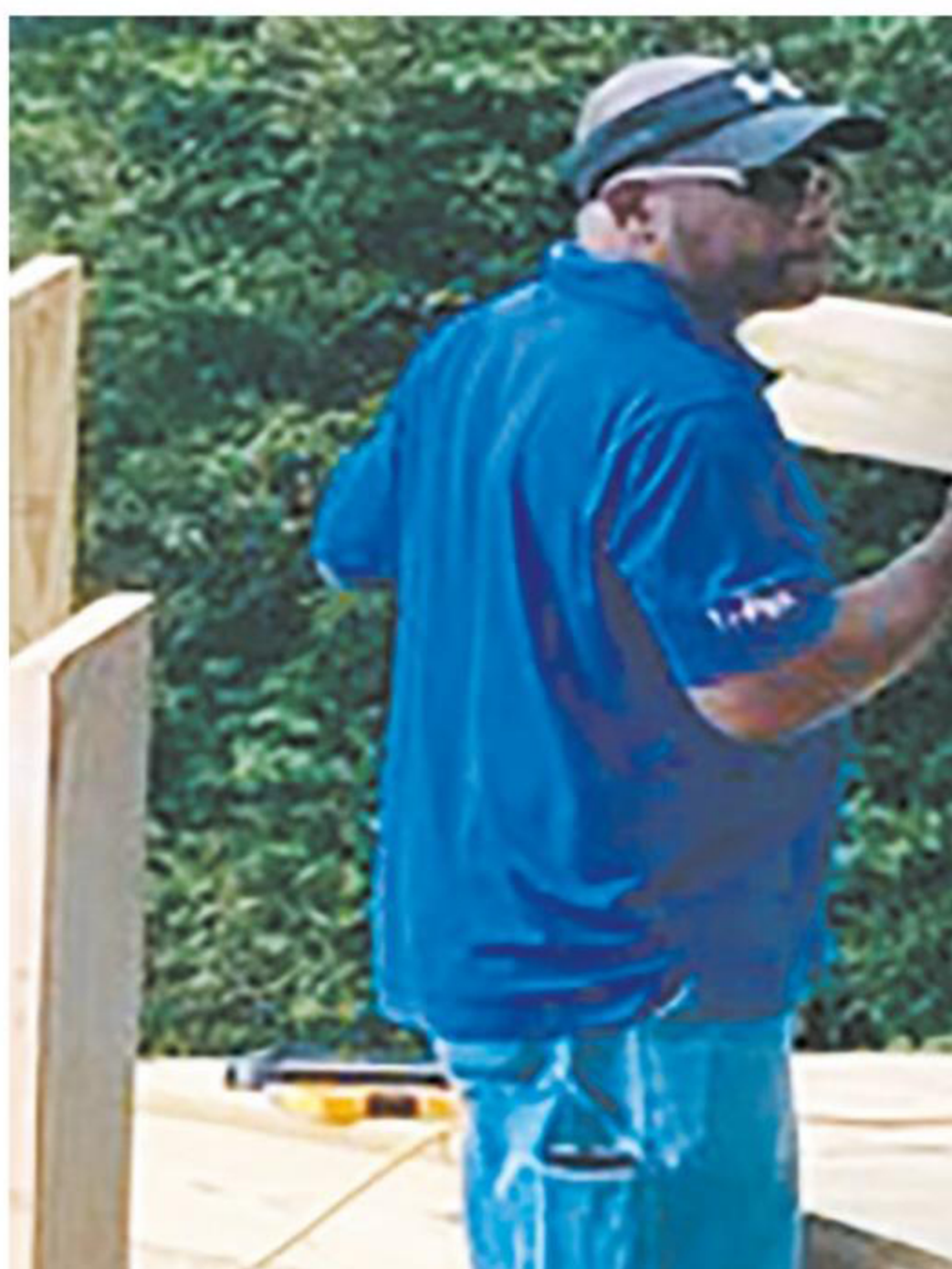
Constructing a wheelchair ramp for a local family.
