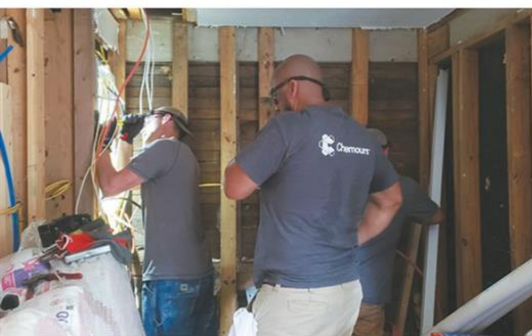
Installing distribution panel.
