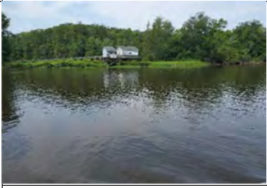
Pump area at kings
