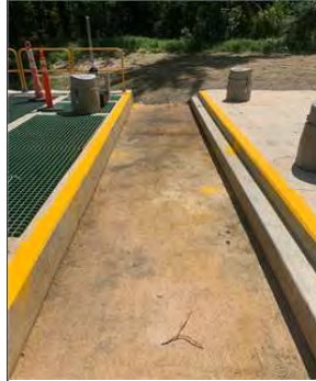
Caption: spillway dry
